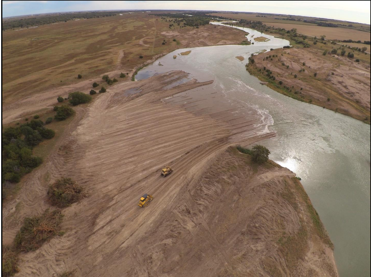
Figure 1.6 Construction of 2019 Sediment Augmentation Project (42,300 yd 3 ).
